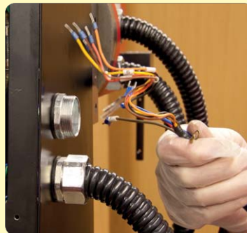
38. Undo gland nut from motor lead tube and pull out motor wires.
