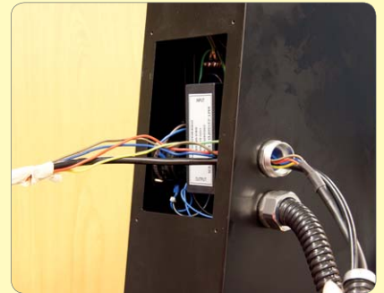
181. Feed wires through side of panel.
