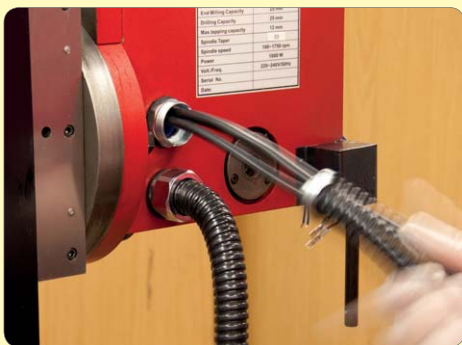
40. Pull lead tube from wires.
