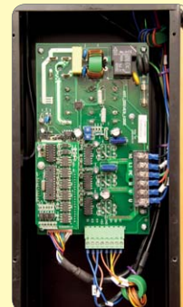
186. The finished panels.
