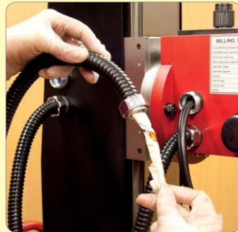
179. Feed wires through lead tube.
