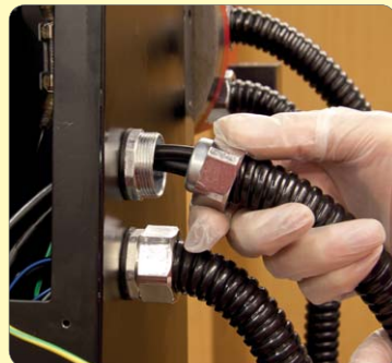
38. Undo gland nut from motor lead tube and pull out motor wires.
