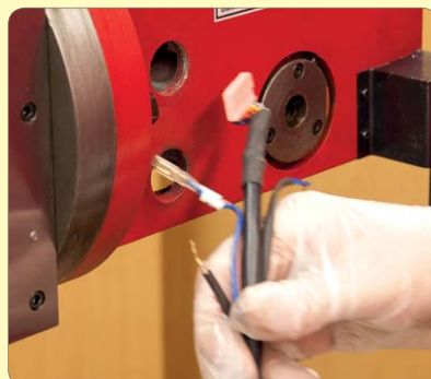
44. Pull out wiring.
